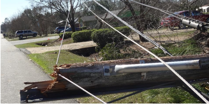
Figure 14: Downed electrical poles snapped throughout the tornado path, many observed with windborne debris. The EF Scale (DI24) gives an expected wind speed of 118 mph for this failure. (Source: UF WHDAG)
