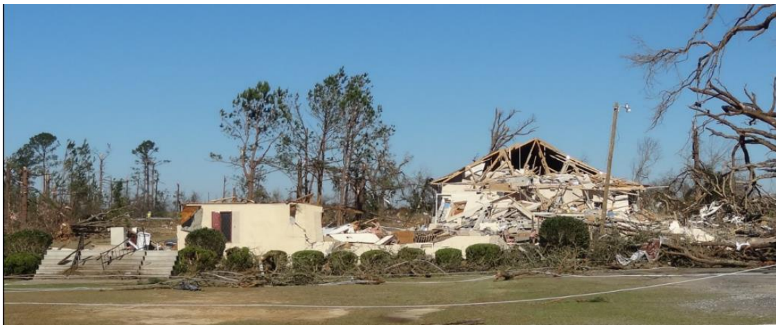
Figure 21: Front view of Albany Baptist Church after the tornado. Nearly half of the new sanctuary was destroyed by the tornado. The older wood-frame sanctuary was completely destroyed except for one interior room.
