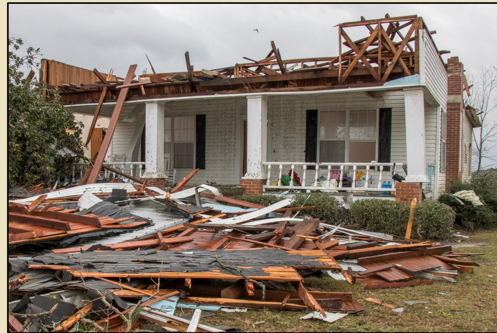
Damage to a 1.5-story residential structure, looking toward the west.
