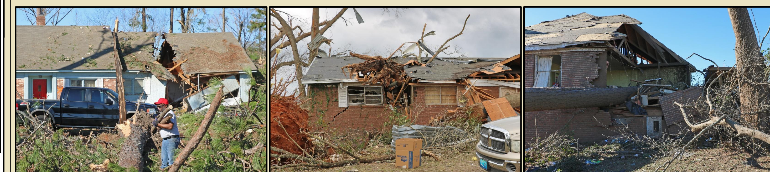
Residential damage following the Albany, GA tornado highlights significant wind-induced tree damage coupled with minor direct wind damage.
