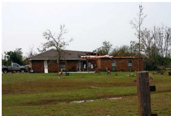
FIG. 6. House with EF2 damage.
