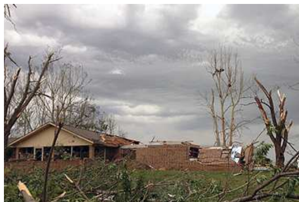
FIG. 8. House with EF2 damage.
