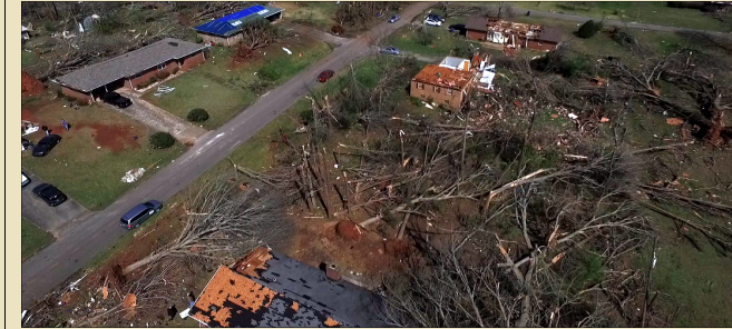
Above: Oblique aerial photograph of tornado damage acquired via drone.
