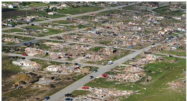
Fig. 14. Tornado Damage in the town of Parkersburg, IA. Most of the town was destroyed by an EF5 tornado on May 25, 2008. Photo courtesy of Iowa Helicopter.
